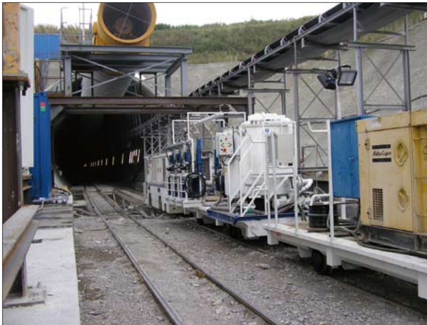
The Wienewald tunnel construction site in Austria. Metax has played a key role in the transportation of cement mixture into the tunnel, providing different types of its injection pumps
